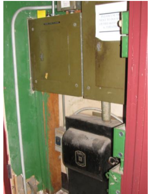
Concessions Panels at Main Lobby
