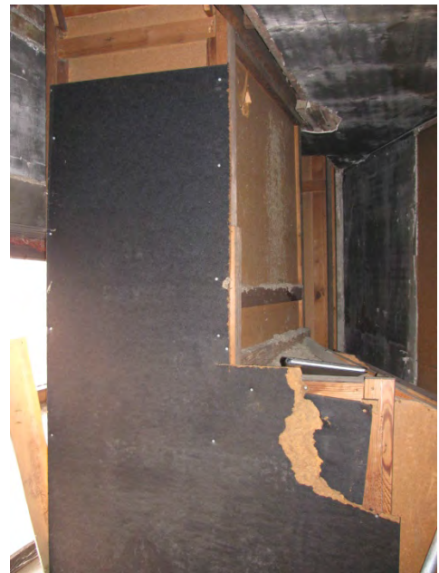
Existing supply duct riser, stage-left
