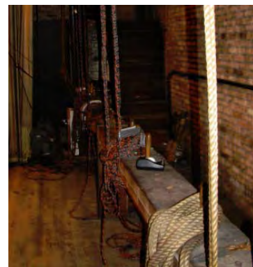
Existing stage right pin rail
