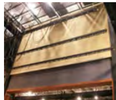
New Brail Fire Curtain System
