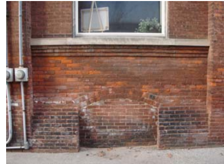
South façade base detail
