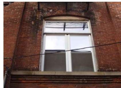
South façade window
