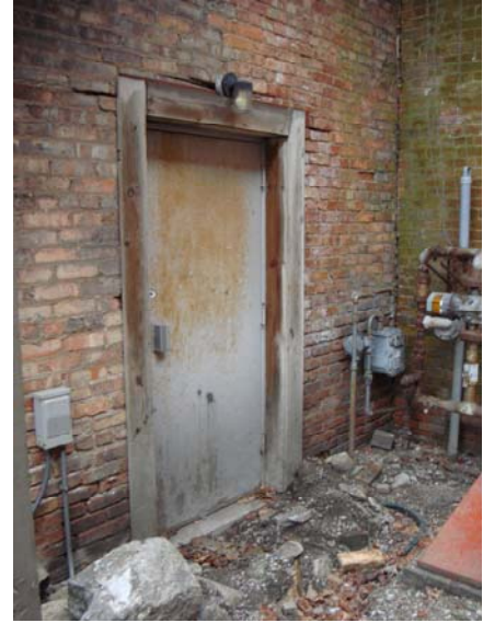
North façade (East entry)
