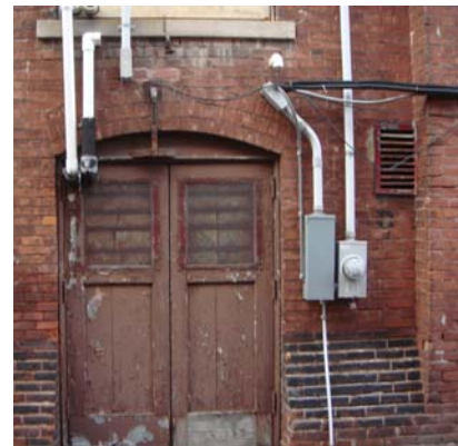
South façade door
